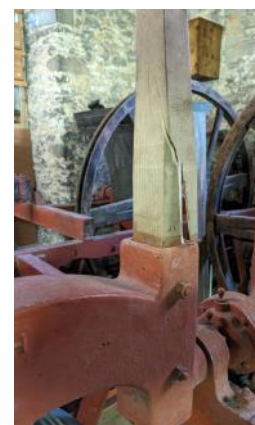
The cracked stay
